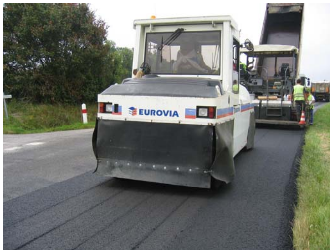
Asphalt application according to DAT Evotherm process
