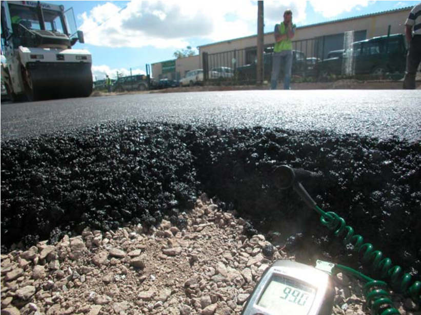
Photo 7: 99°C temperature during compacting
