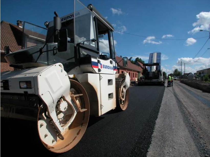
Photo 7: 99°C temperature during compacting
