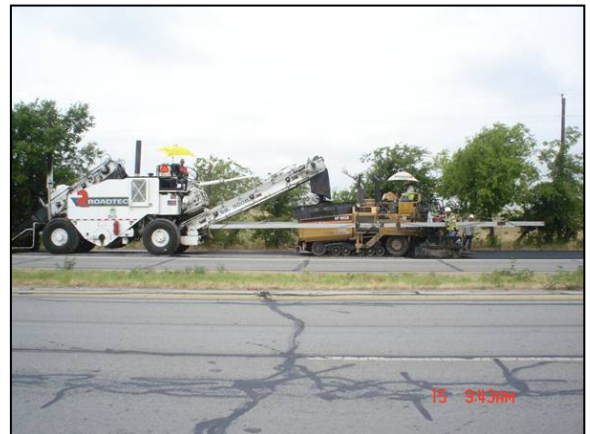
Sealed Transverse Cracks on Existing Pavement
