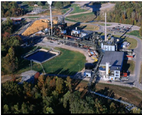
WICKLIFFE, KENTUCKY CARBON MANUFACTURING PLANT
