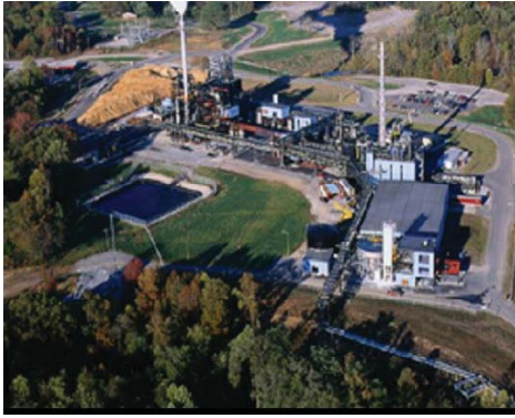
WICKLIFFE, KENTUCKY CARBON MANUFACTURING PLANT
